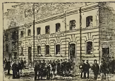
THE MISSIONS TO SEAMEN CHURCH AND INSTITUTE, WELL STREET, LONDON DOCKS, E.
